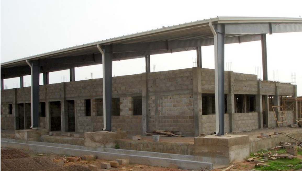
3 rd Wing under construction
